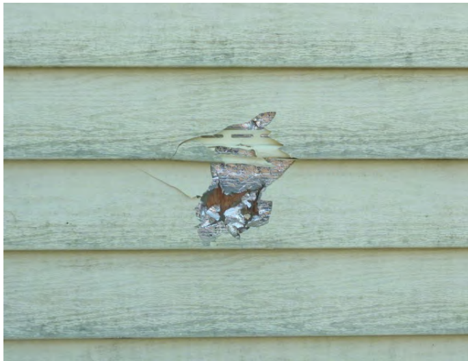
Typical damaged vinyl siding at numerous locations at each building.
