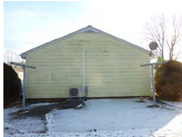
Typical side, front and rear elevations have staining.
