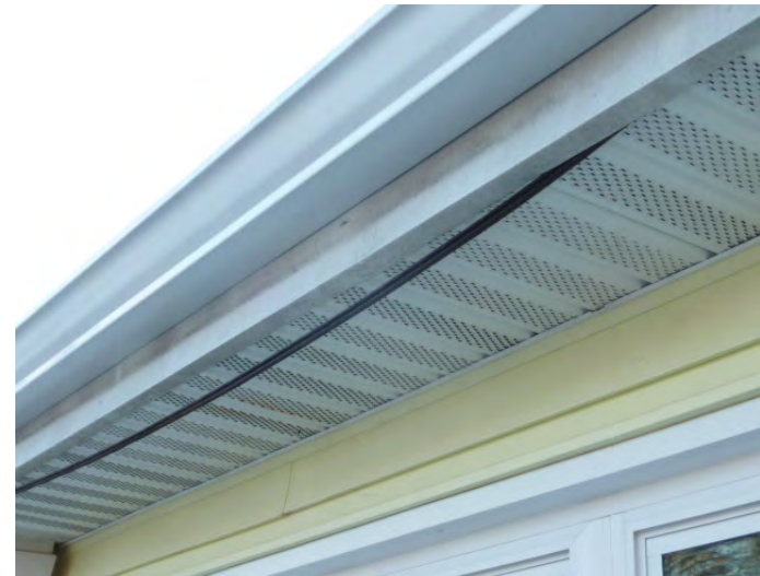
Fascia behind gutter has staining and the soffit gasket is displaced at select locations.
