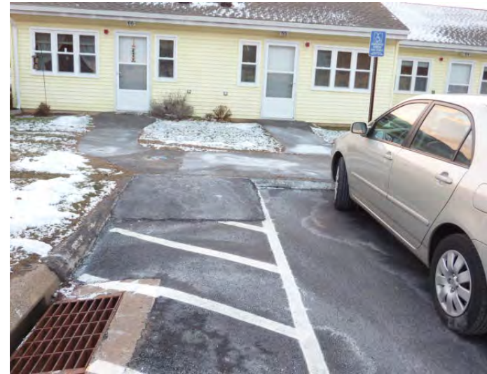
Sloped asphalt patch to improve an accessible route. Striping is scheduled for the spring.
